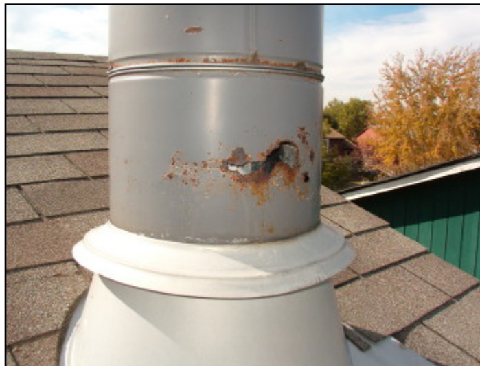
13. Rusted chimney wall from fireplace
