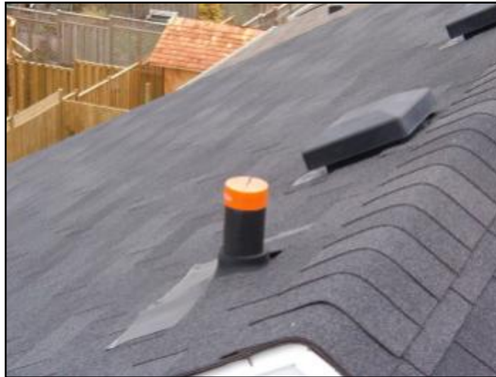
18. Plumbing stack is capped
