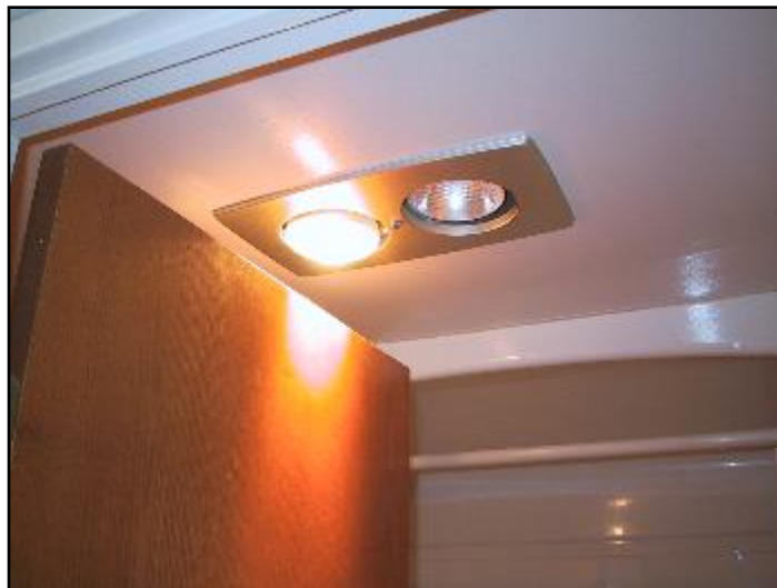
8. Heat lamp over door - fire hazard!
