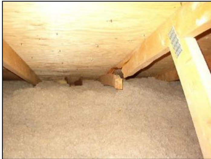
5. Top chord of truss is broken
