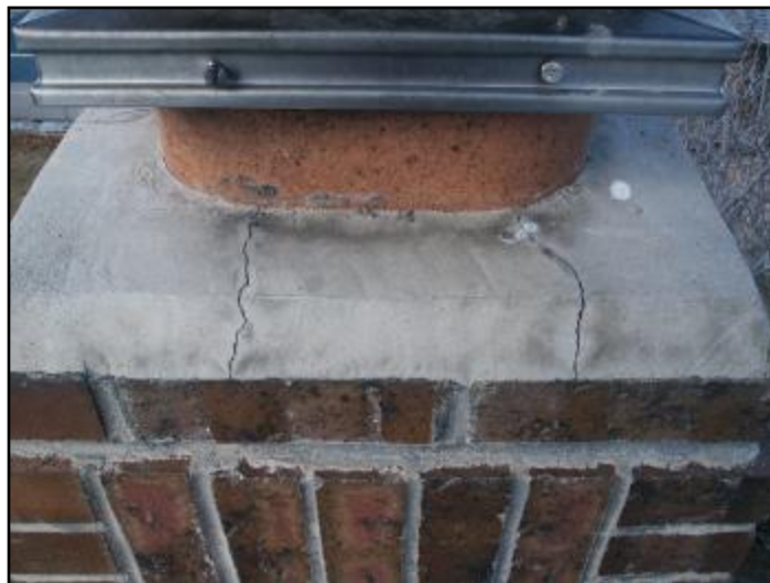
12. Minor cracks in chimney cap
