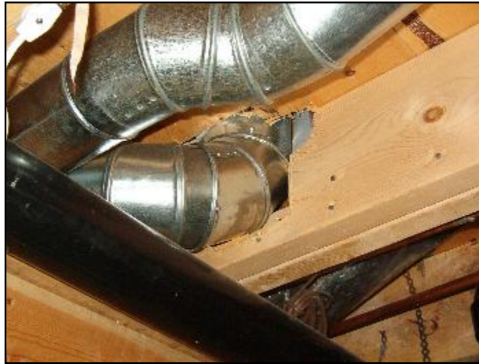
4. Double joist cut for ductwork
