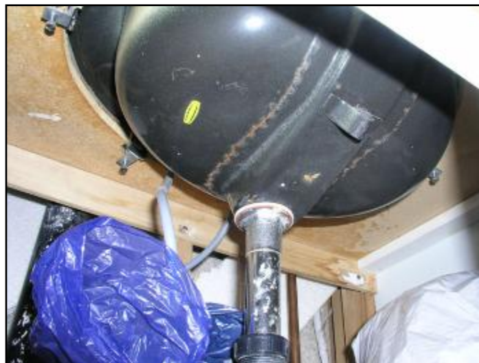
19. Steel basin rusting at weld
