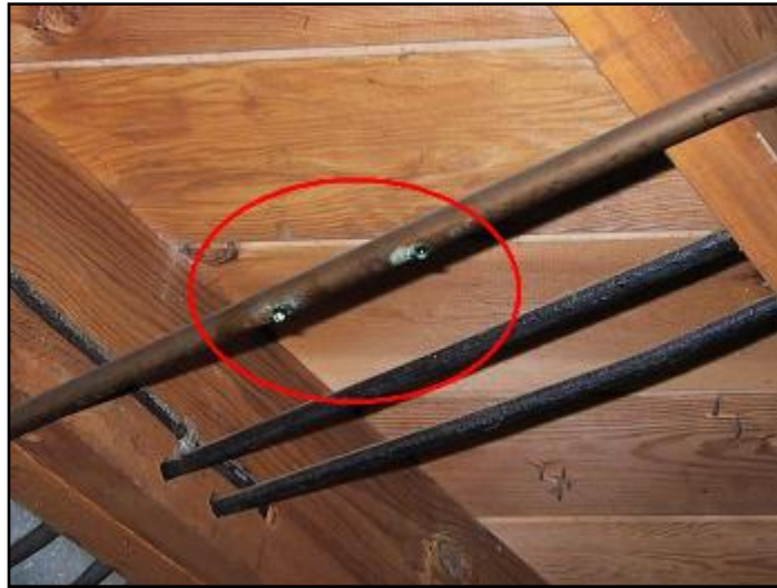
16. Leaking copper supply pipe
