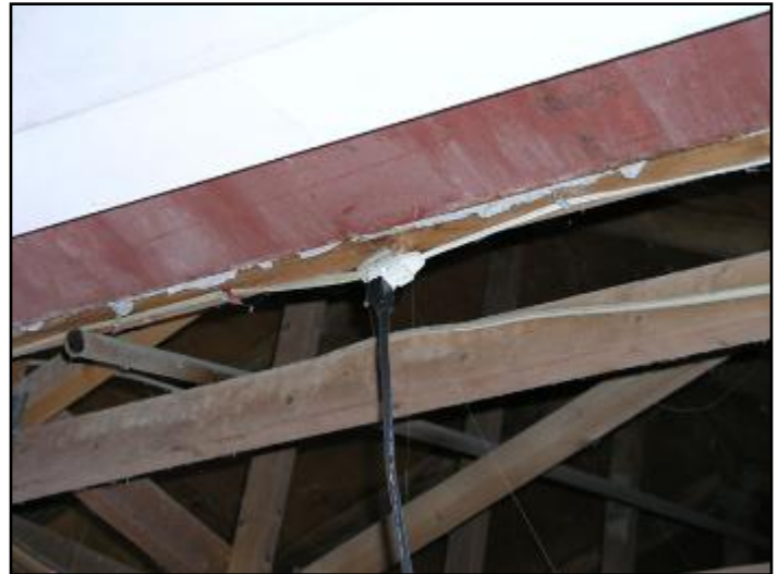
21. Extension cord for east garage door opener
