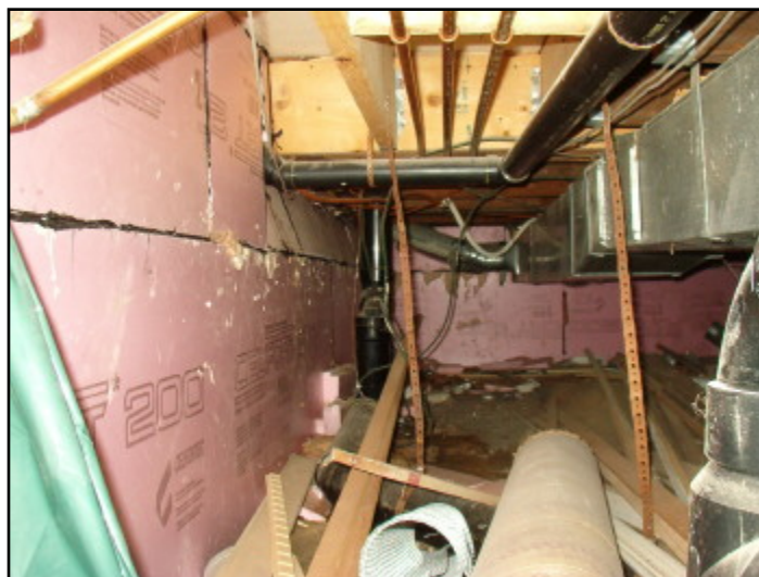
15. Exposed polystyrene insulation is fire hazard
