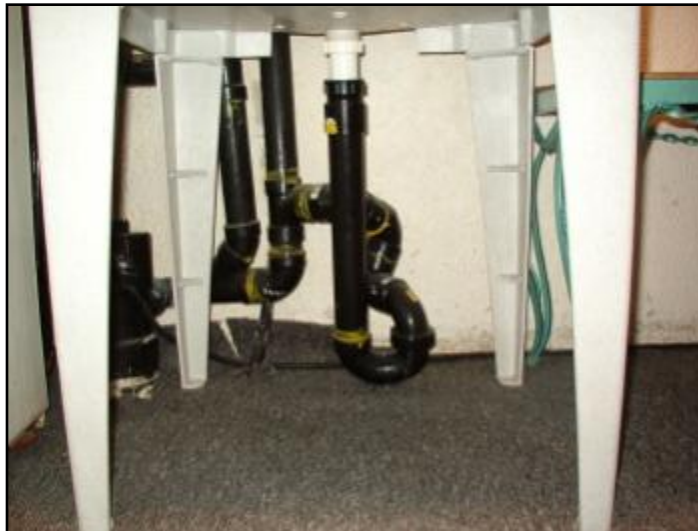
17. Poor trap arrangement
