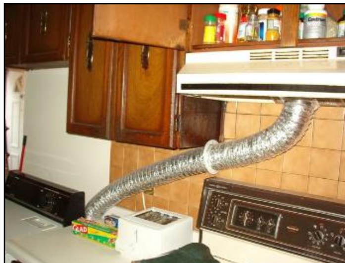
22. Clothes dryer vented incorrectly
