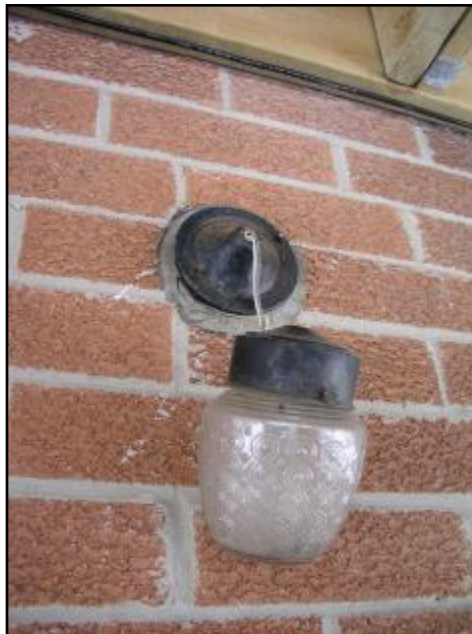
7. Light fixture is not well secured
